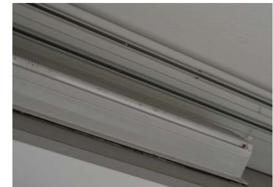
Hard plastic element with rails milled into the surface, used to hang the curtains, installed later on.
