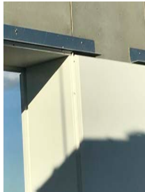
Steel Brackets supporting cladding
