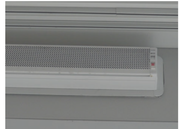
Outlet- ventilation unit on the interior
